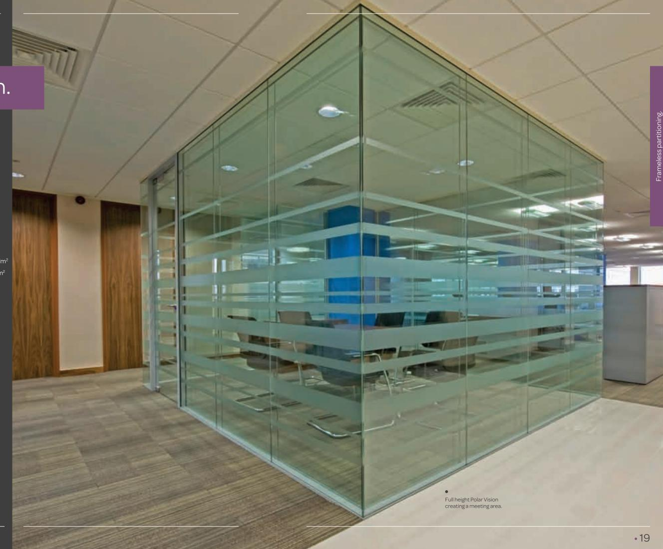
A truly integrated and versatile solution combining single glazed, double glazed and solid elements.
