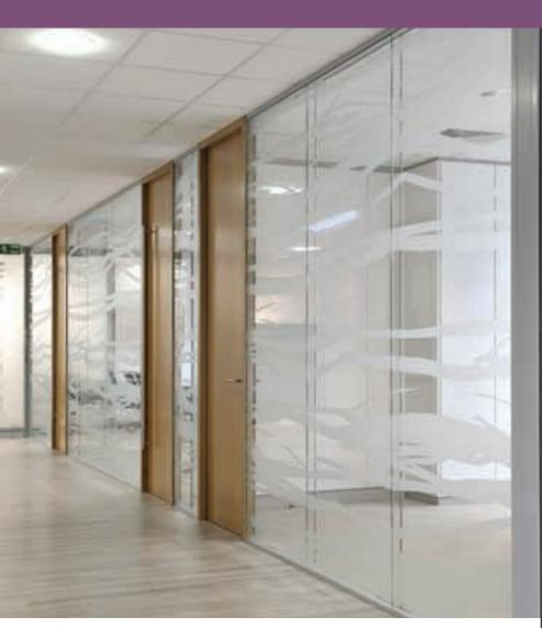
Polar Vision is dry jointed and constructed without mullion posts, offering up to 30 mins fire protection for both integrity and insulation.
